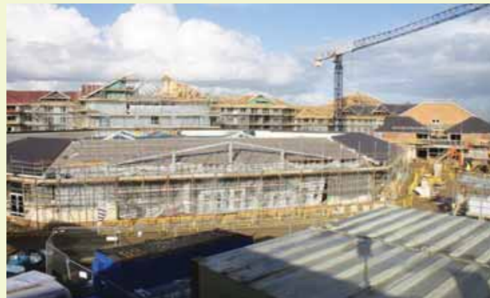
Construction – less than a year to go
