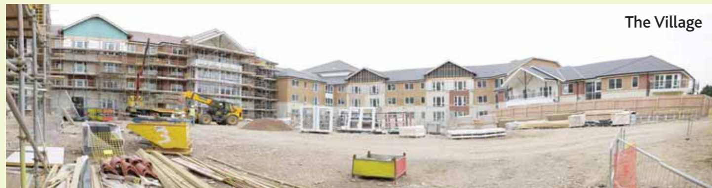
Balconies are being installed
